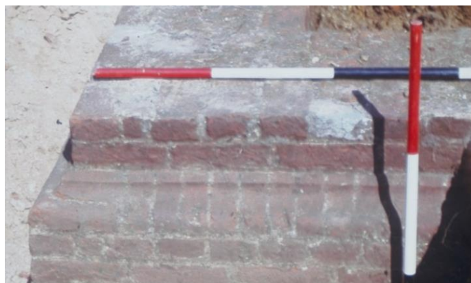
Pl. 37: Tr. B, Moulded Brick Plinth at the South West Corner of Tower [125], Looking North East
