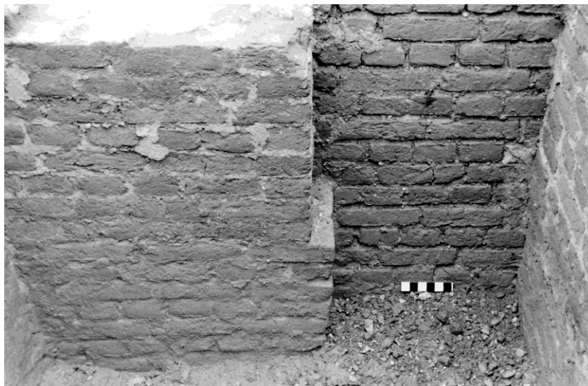
Pl. 44: Tr. H/I/J, Smaller Tower [116], Looking South East
